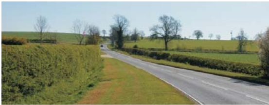
Nobottle Road looking east from Whilton Locks towards Whilton village
