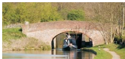
Bridge 14 and lock gates, Grand Union Canal
